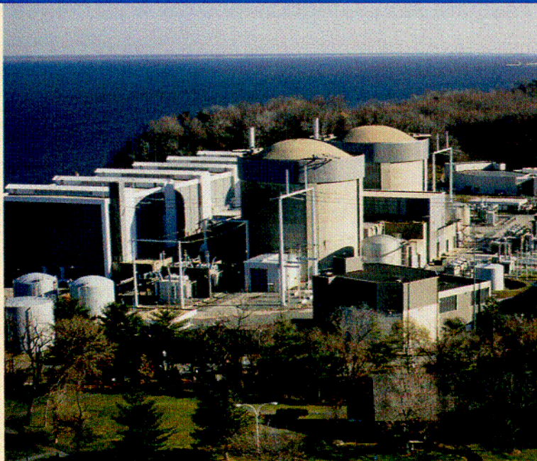
In March 2000, Constellation Energy's 1,700-megawatt Calvert Cliffs Nuclear Power Plant on the Chesapeake Bay became the first nuclear facility in the country to have its operating licenses renewed. The plant's two units now have 20 additional years of operating life through 2034 and 2036.
