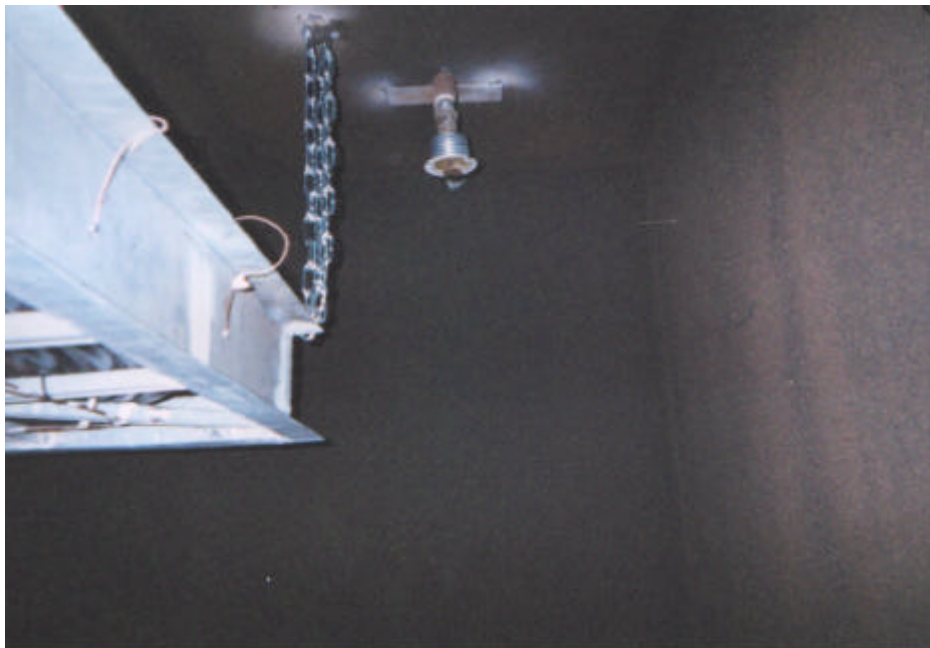
Figure 4-7. Water sprinkler head inside fire test cell.
