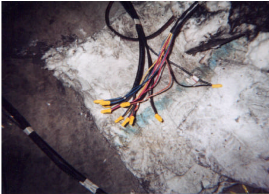
Figure 3-11. IR Measurement system "In" wiring harness connection to the test cable bundle.
