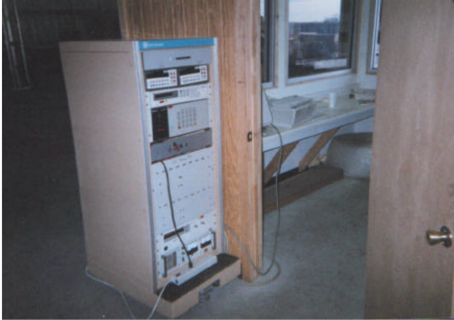
Figure 3-9. Front view of the IR Measurement system instrument rack.
