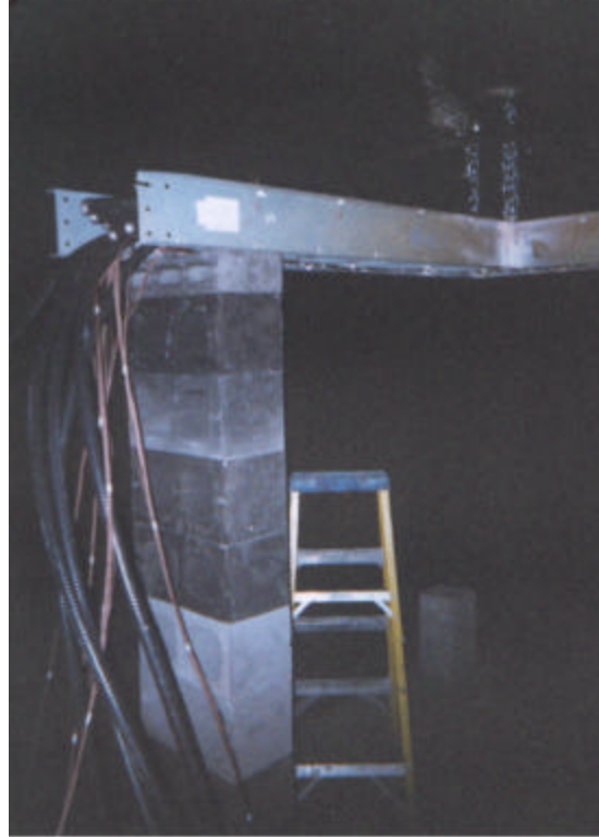
Figure 4-4. Tray, with cables, installed in fire test cell.
