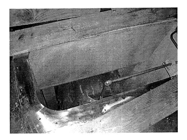
This picture shows the general configuration of the sand-box areas for Farley-1 and -2. The Reactor Coolant system piping can be seen in the middle of the picture. Sufficient space exists for an individual to stand next to the piping but movement is very limited. Farley will use a video camera to perform a general visual examination of the accessible support structure and associated components.
