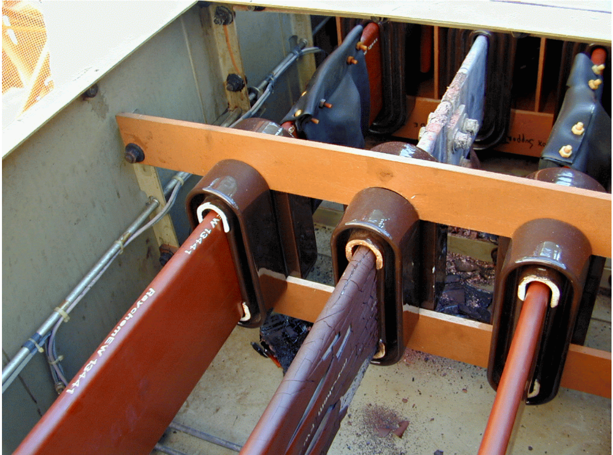
View 1 of BUS 309 Showing degraded Insulation on Bus Bar
