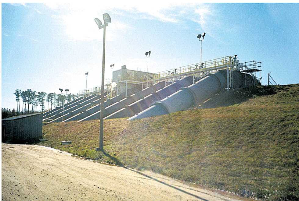
Pipes at low-level intake move water from the James River (on the left), over the canal dike, and into the canal (on the right).
