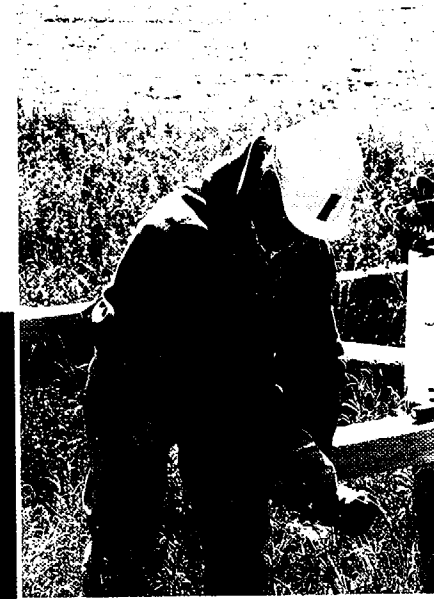
Bob Nielsen, line foreman, assembles a cross arm on a pole used in rebuilding a line near Alta.
