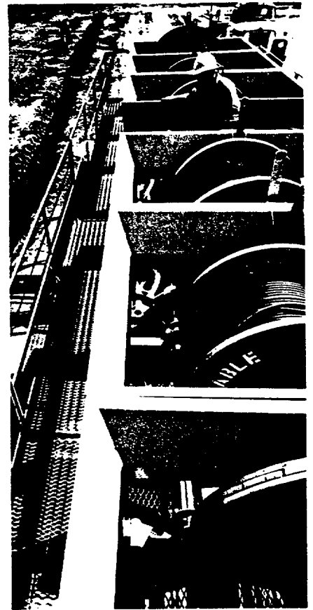
A cable-laying machine, designed specifically to lay the Westinghouse-developed electronic "nervous system" for San Francisco's Bay Area Rapid Transit System, unreels some of the 800 miles of cable that will be needed for the 75-mile system.
