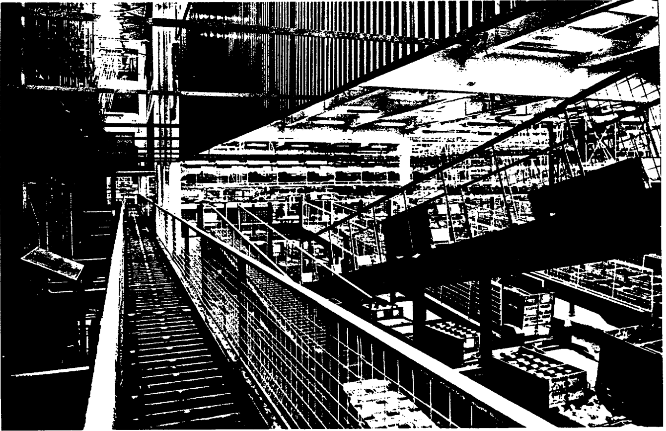
The largest computer-controlled warehouse in Europe is under construction in Sweden for a major truck and bus manufacturer.
