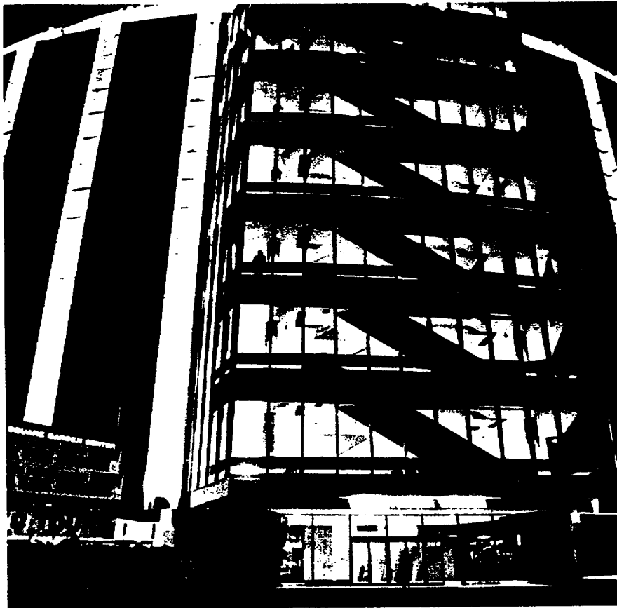
Forty-eight Westinghouse electric stairways serve the new Madison Square Garden. Each four-foot-wide stairway, traveling 120 feet per minute, can move 9,200 passengers an hour.
