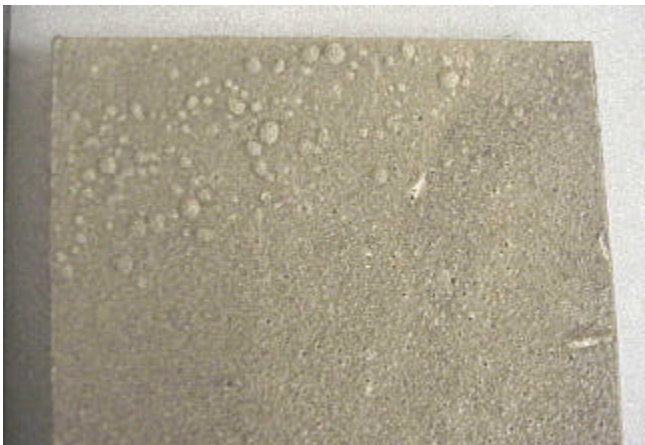
Figure 3-23. Detail of the surface of the irradiation-aged specimen after DBA testing. Note the presence of intact blisters in the coating.
