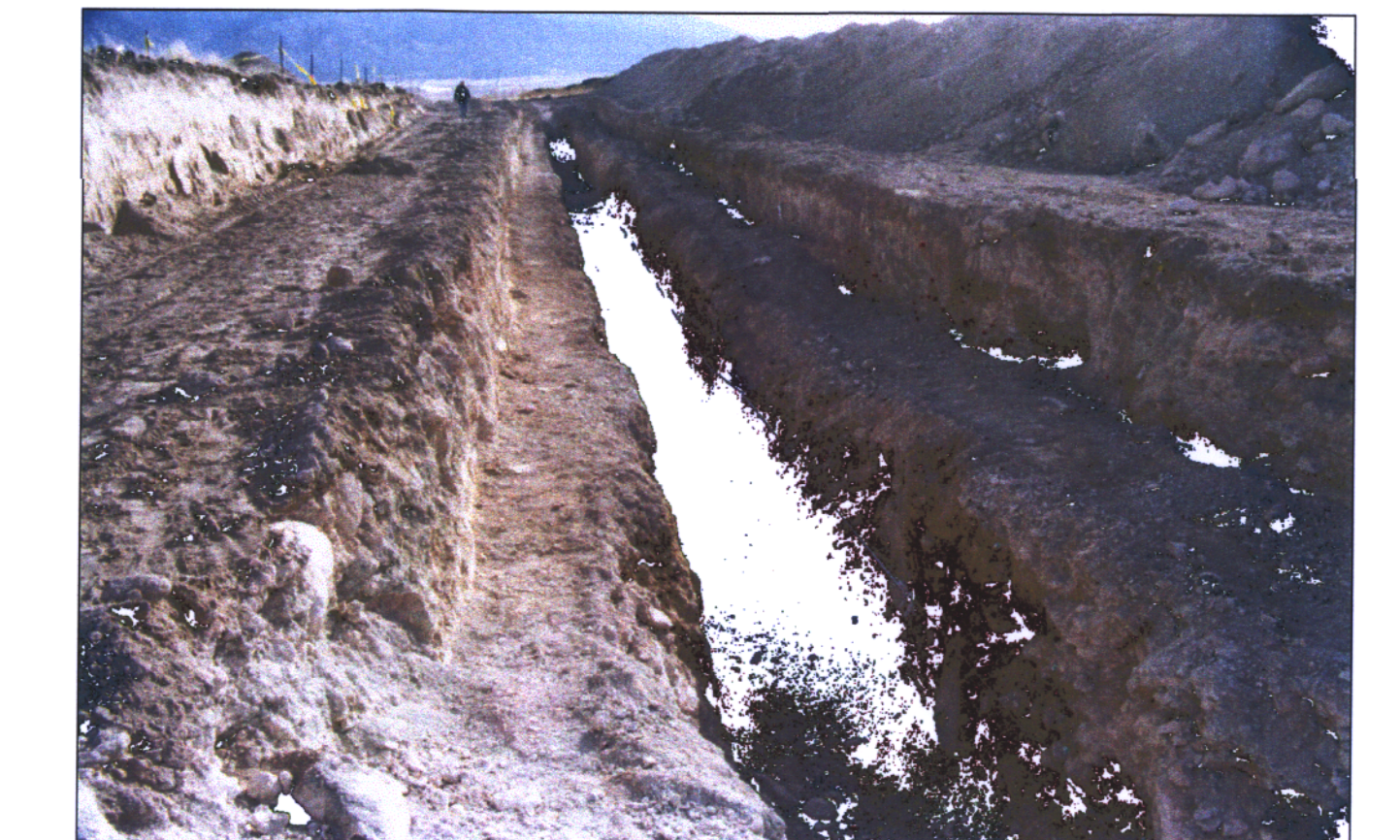
Trench T-1, view looking east
