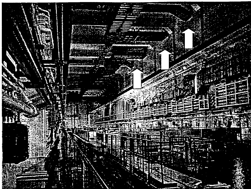
Figure F-5 – FHB HVAC Penetrations
