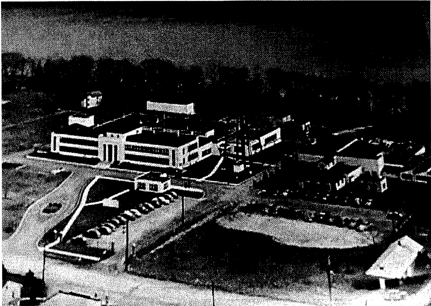
Figure 2-1 Safety Light Facility
