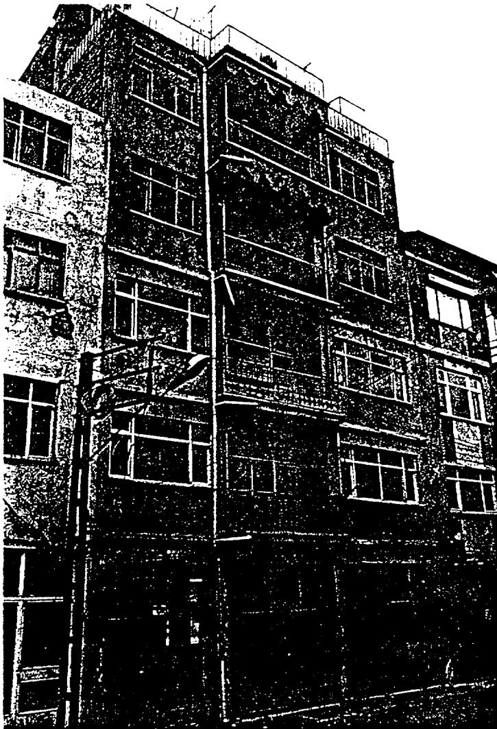
Fig.19. Medium damage in a five story reinforced concrete frame due to soft ground story.
