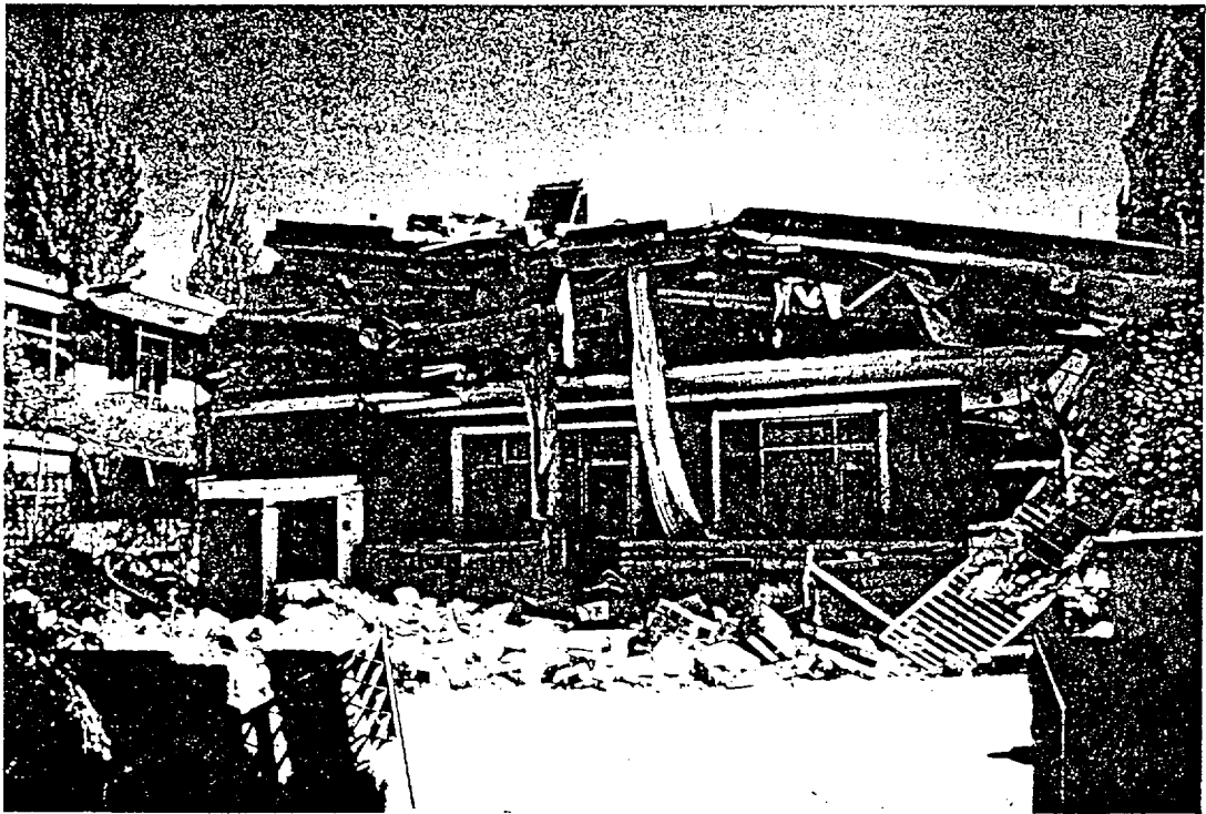
Fig. 17. Three story masonry building having identical failure pattern with the building in Fig. 16. The original first stories sustained light damage in both buildings.
