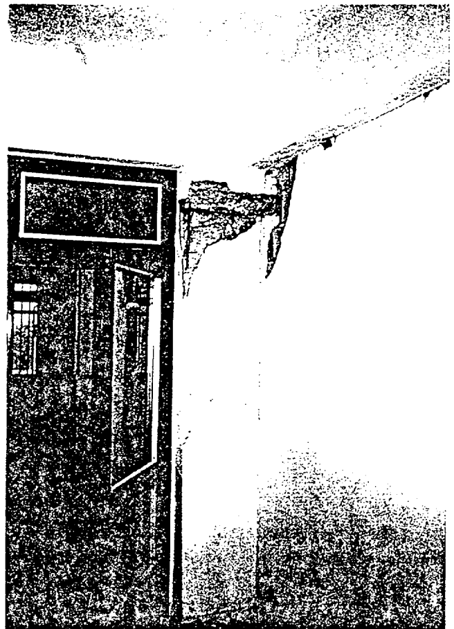
Fig.23. Shear-flexure failure in a weak column connecting to stronger beams. Notice inadequate spacing of stirrups.
