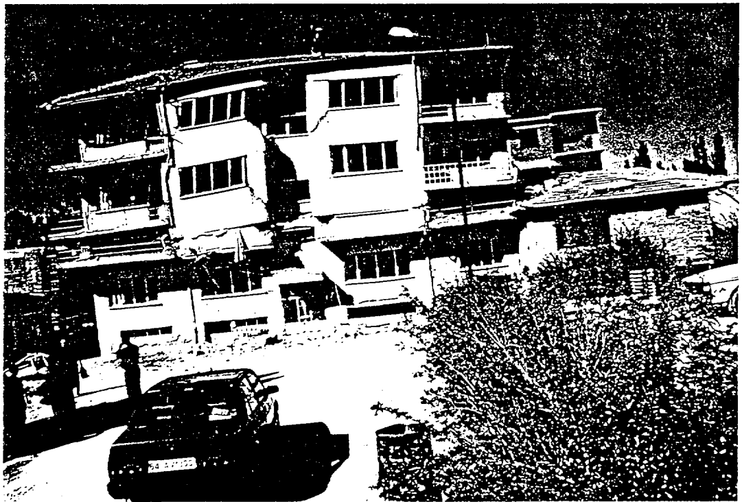
Fig.15. Middle story failure due to pounding.
