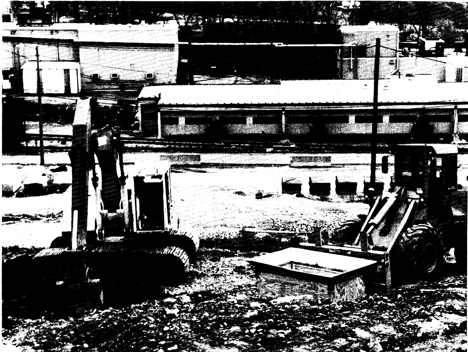
Photo 6.1. Low-level radioactive soil being loaded into boxes at the Mound Plant. (Courtesy of EG&G Mound Applied Technologies, Miamisburg, Ohio, and the Hazardous Waste Remedial Actions Program, Oak Ridge, Tennessee.)
