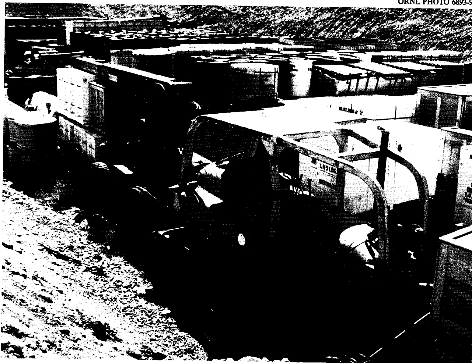
Photo 4.1. Placement of waste in a low-level waste burial trench at the Hanford Site. (Courtesy of Westinghouse Hanford Company, Richland, Washington, and the Hazardous Waste Remedial Actions Program, Oak Ridge, Tennessee.)
