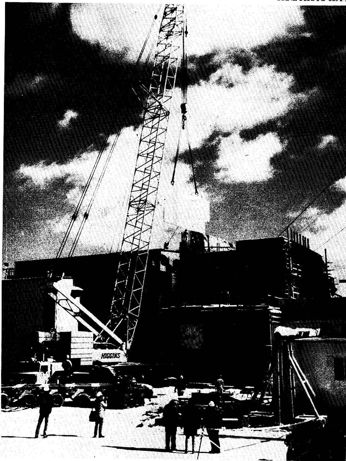
Photo 2.1. Construction of the West Valley Demonstration Project vitrification facility that will incorporate West Valley high-level waste into a glass. (Courtesy of the DOE West Valley Project Office, West Valley, New York.)
