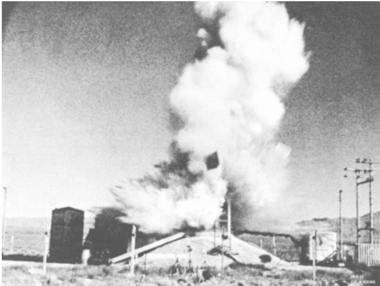
Figure 59. The destructive excursion in BORAX, 22 July 1954.
