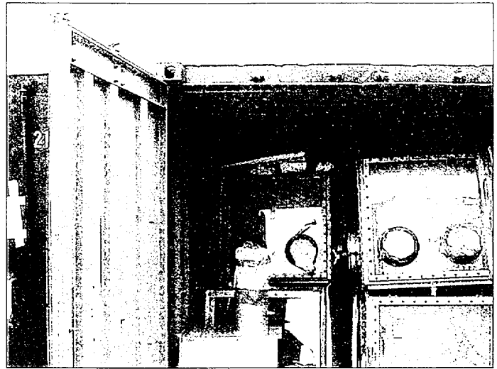
Gloveboxes and fume hoods headed for supercompaction.
