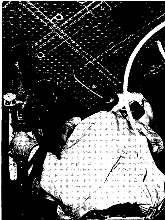
FIGURE 3.25. Tube Pulling Through Tube Sheet; Hydraulic Jack in Operation
