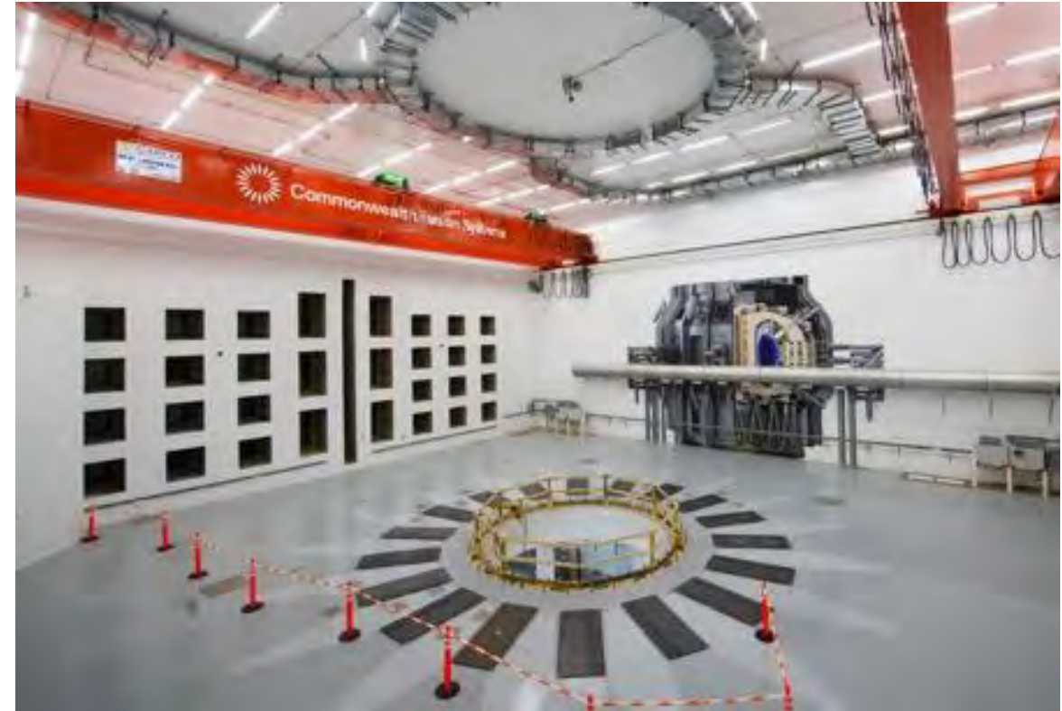
SPARC Tokamak Hall under construction in Devens, MA
