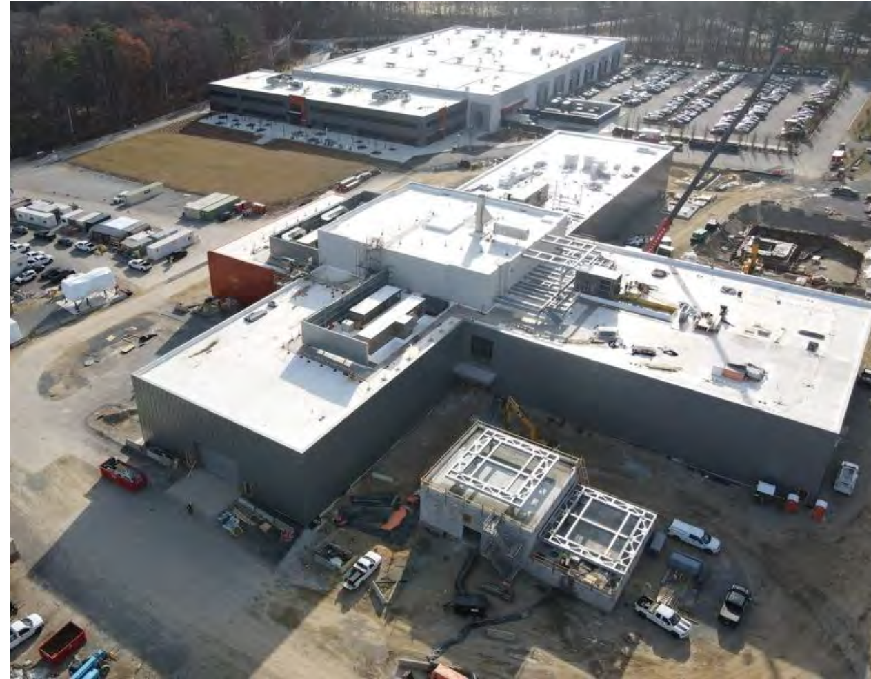
SPARC under construction in Devens, MA
