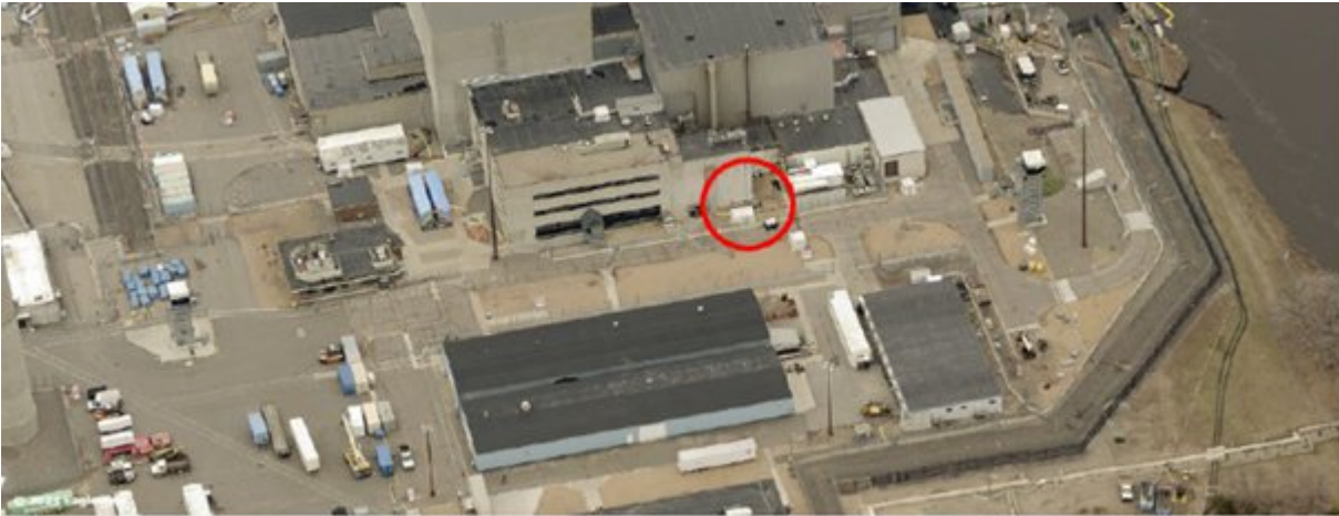
Figure 1 – Side View of the Approximate Spill Location on May 21, 2023.
