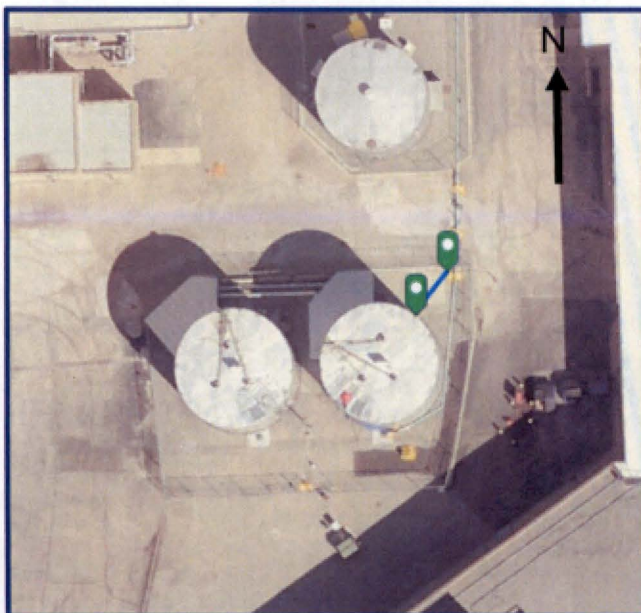
Figure 3: 2/3 Condensate Storage Tanks
