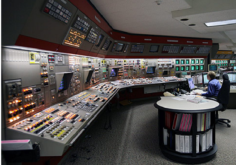
Figure A-1 Example of a full-scale MCR training simulator for an NPP
