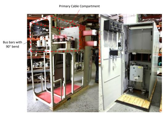
Figure 4-1 GE Type M-36 switchgear enclosure
