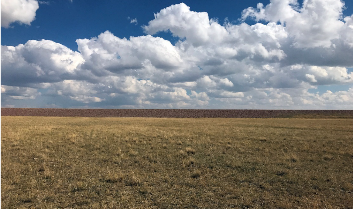
Figure 6-17 Surface and Vegetation Condition on the Disposal Cell at Shirley Basin South, Wyoming
