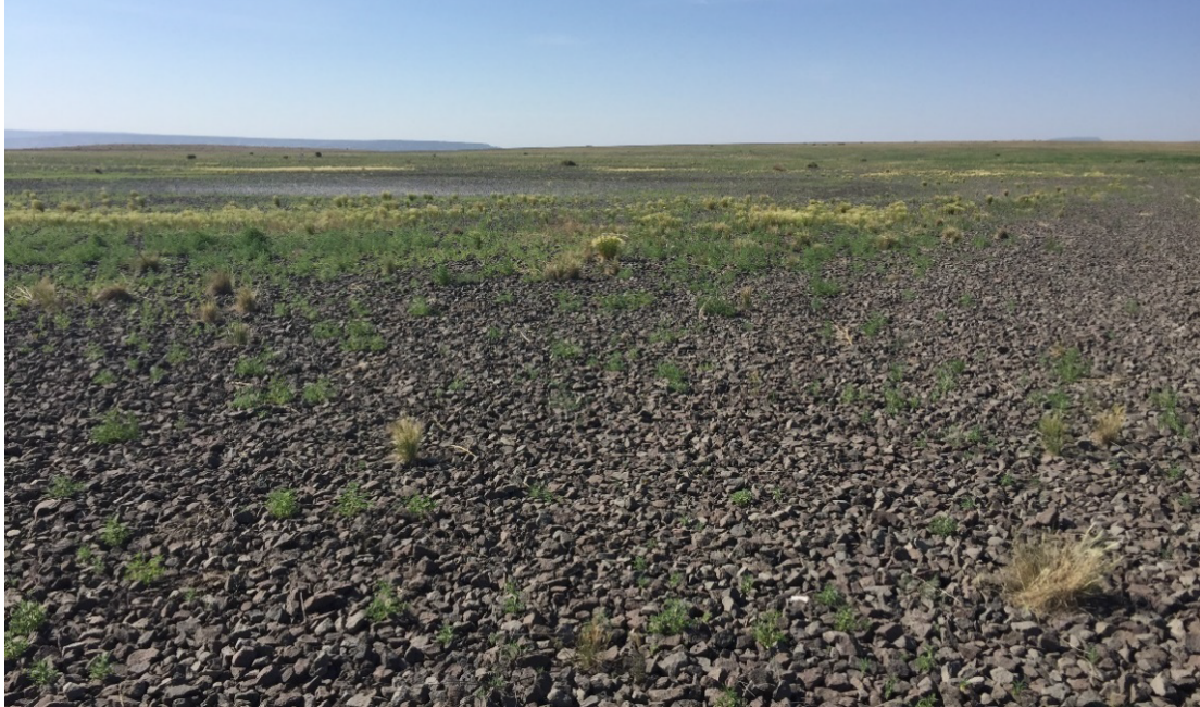
Figure 6-10 Surface and Vegetation Condition on the Main Disposal Cell at Bluewater, New Mexico
