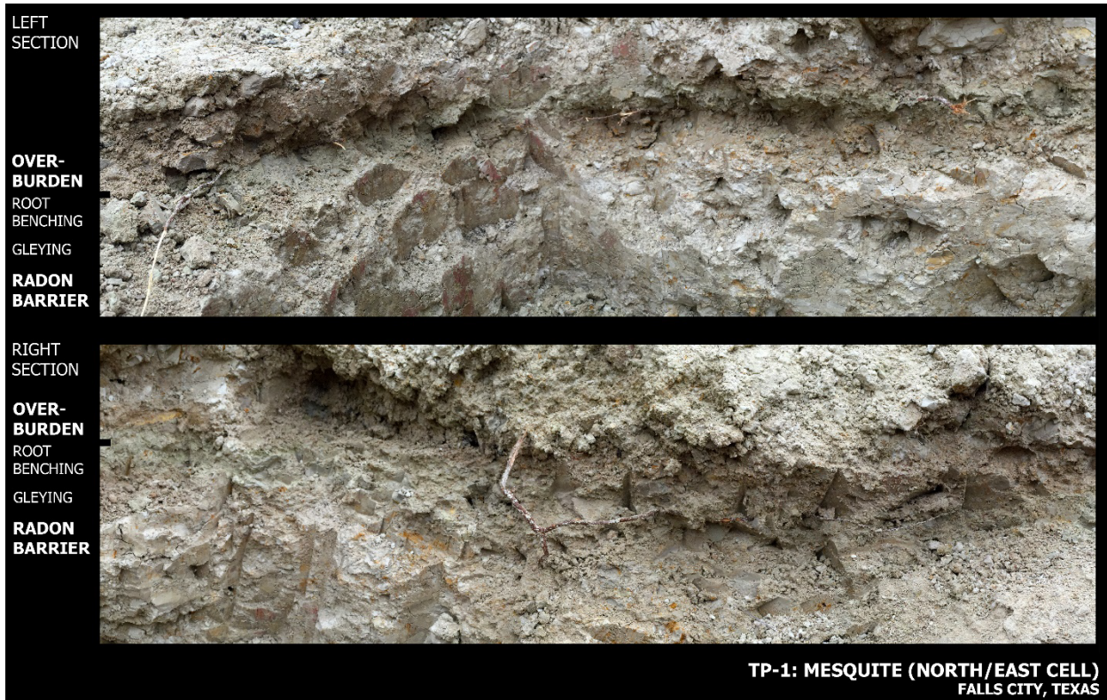
Figure 6-7 Honey Mesquite Root Benching and Gleying Along the Top Boundary of the Radon Barrier at Falls City, Texas
