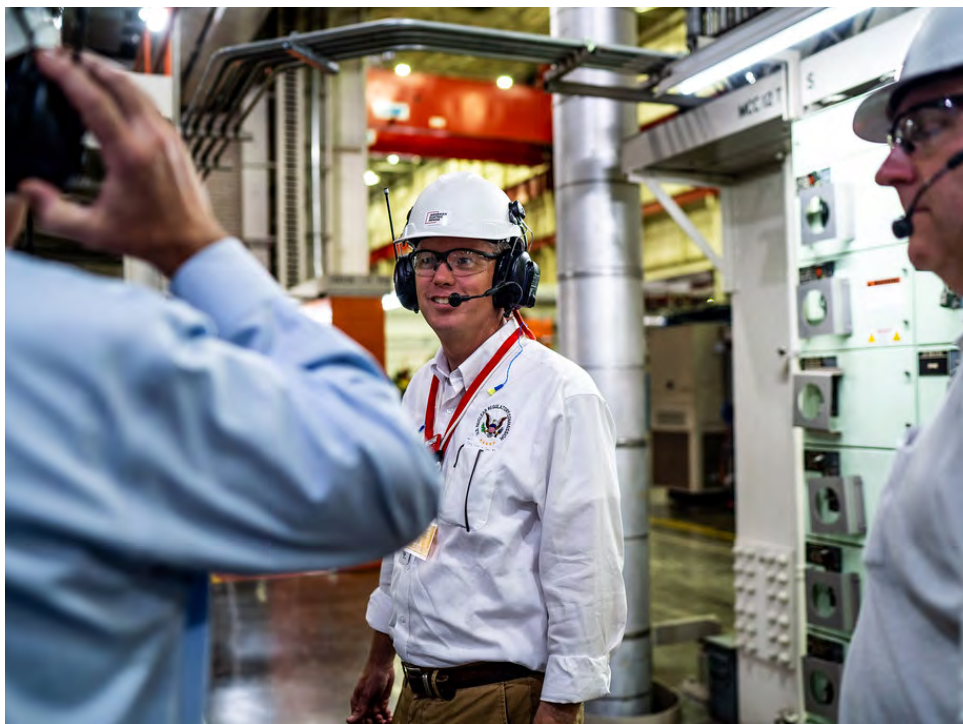
NRC Chairman Christopher Hanson tours the Donald C. Cook nuclear power plant and talks to licensee staff during a facility visit. Photo courtesy of Indiana Michigan Power.
