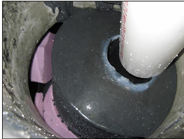
Figure 5-17 Dislodged Penetration 5.2
