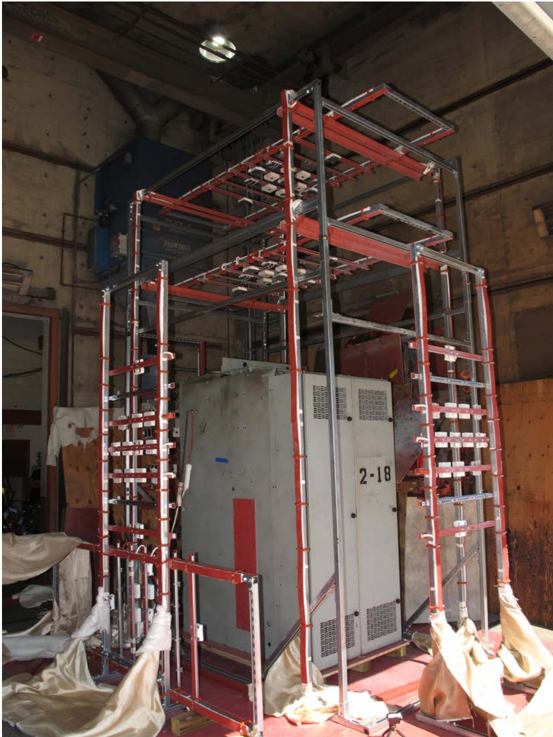
Fig. 31. Photo of Instrumentation Racks for Test 2-18A Test 2-18B.
