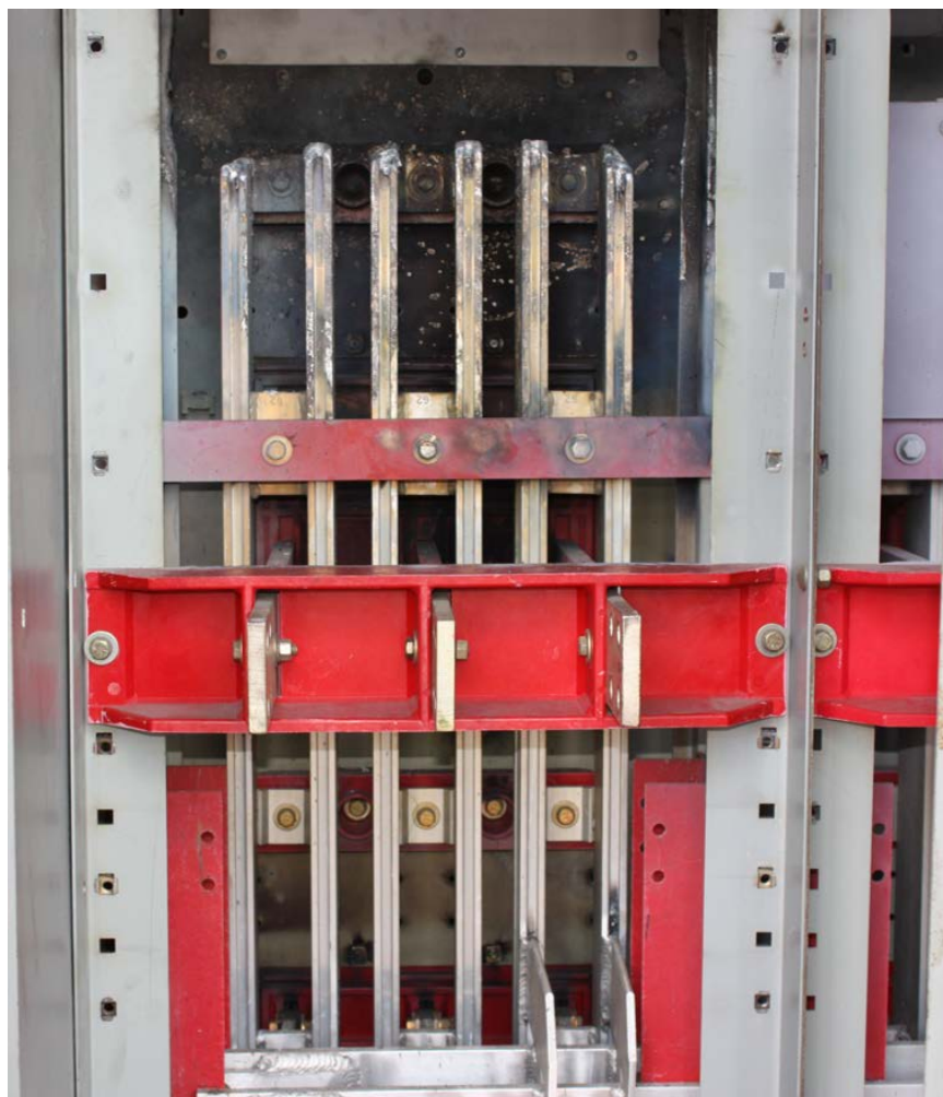
Fig. 54. Main bus bar post-experiment.
