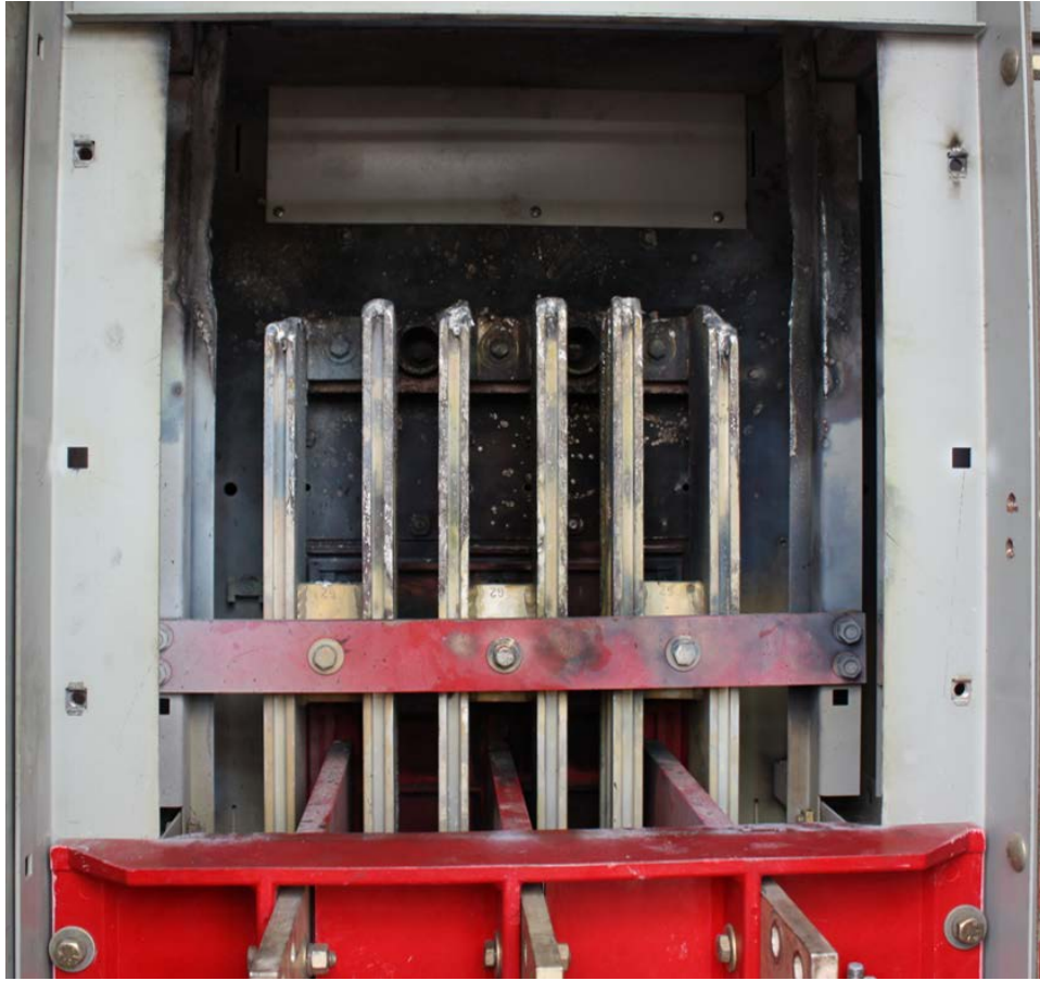
Fig. 46. Enclosure Post-Test 2-13D.
