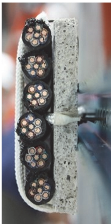
Fig. 23. Cable coupon constructed of seven conductor PE / PVC control cable (Cable 900). Side view.
