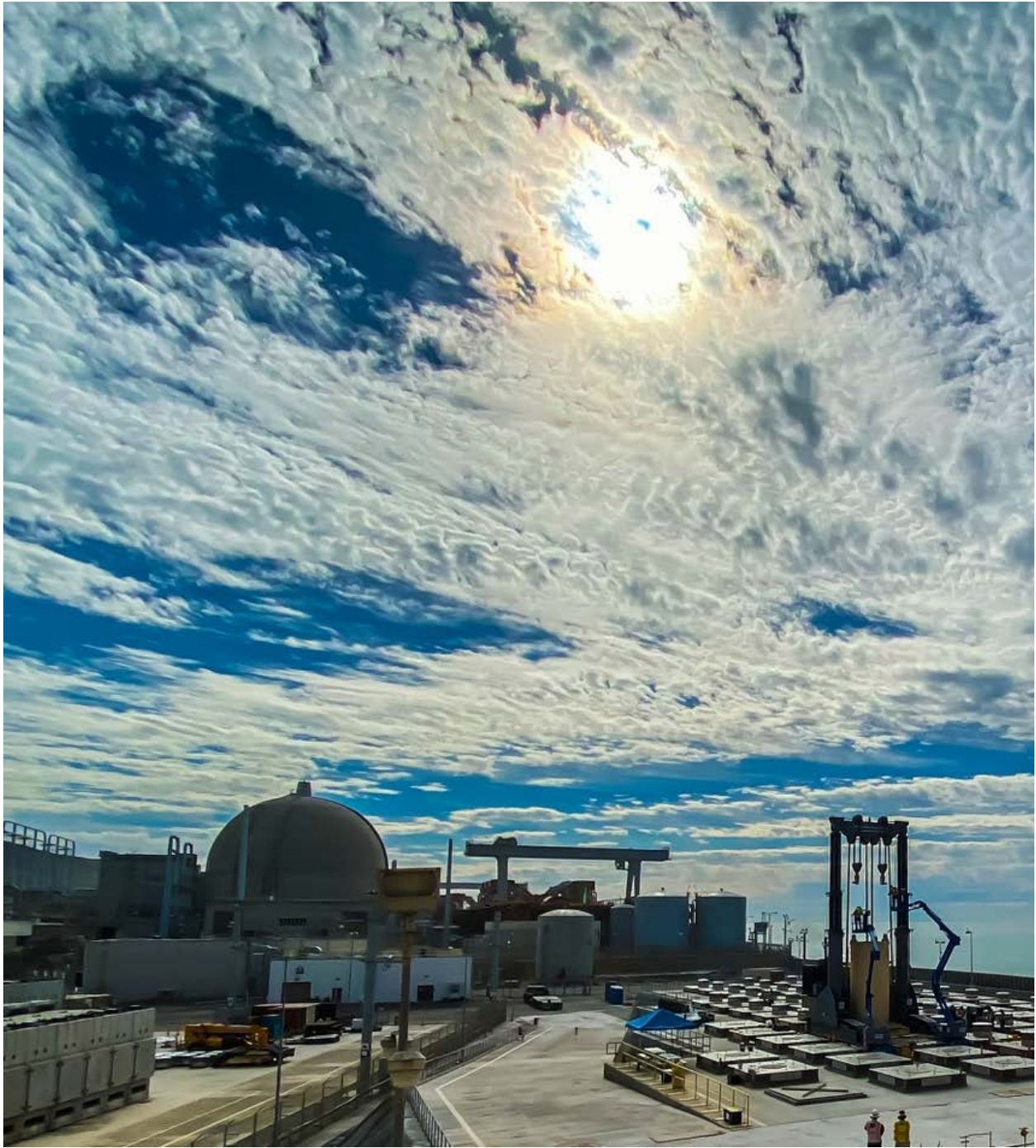
Fuel transfer operations at SONGS
