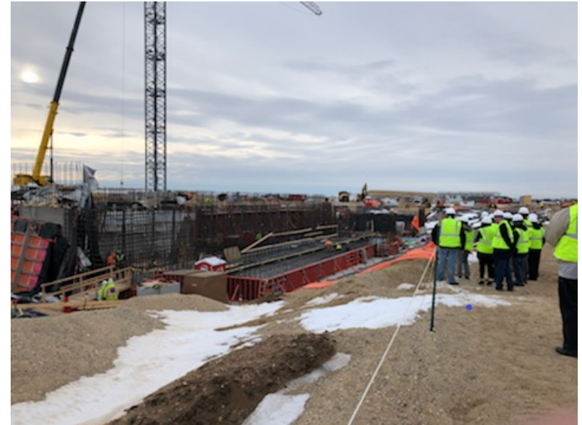
SHINE Construction Site in February 2020
