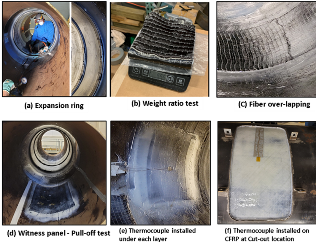
Figure 21 Some other steps in CFRP repair installation process
