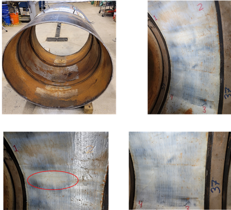
Figure 34 River-like matrix cracking on CFRP system inside the pipe after hydrostatic test
