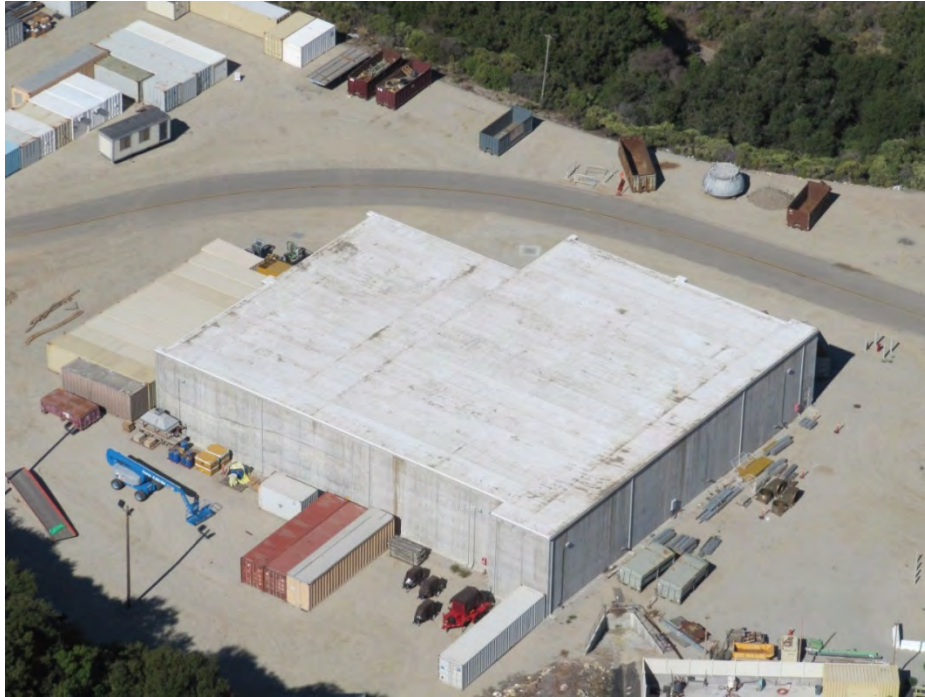
Old Steam Generator Storage Facility looking northwest
