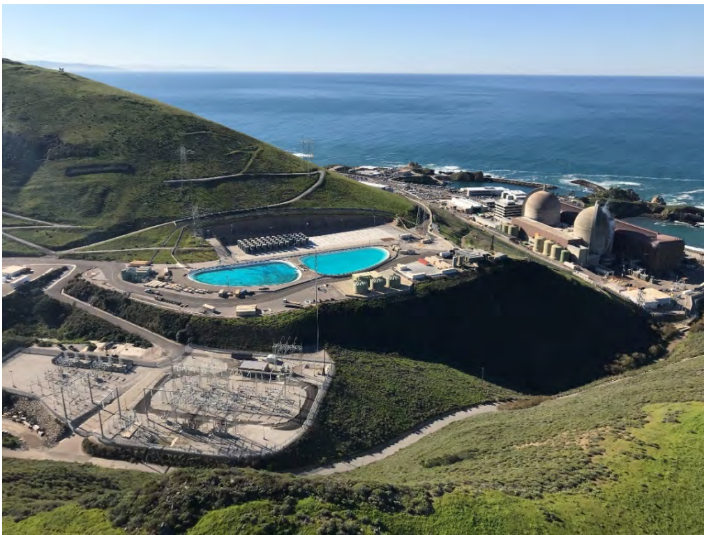
DCPP ISFSI Pad within hillside, on south side of the make-up water reservoirs
