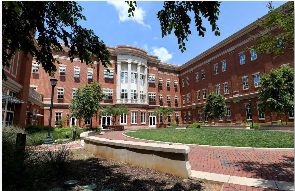
Albert and Freeman Energy Production and Infrastructure Center
