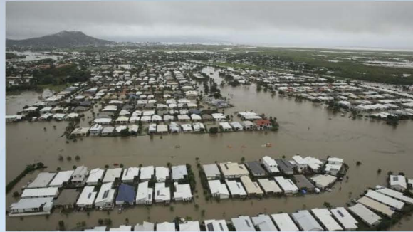
Townsville flood, January 2019 Photo: Courier Mail USD$4 billion damages
