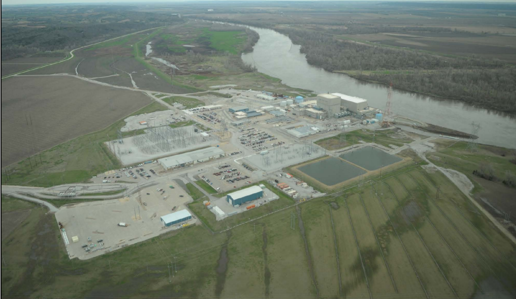
Before (Looking North)
