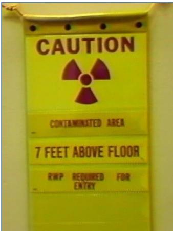
A radiation work permit was required to access contaminated ceiling areas above the clean lower areas of the auxiliary building main corridors.
