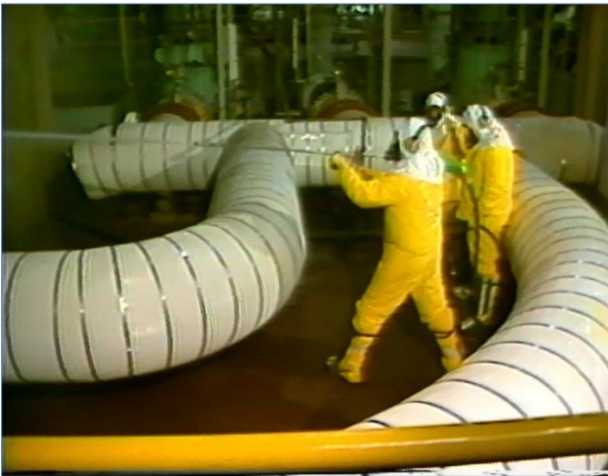
Decontamination using a high-pressure hydrolance.
