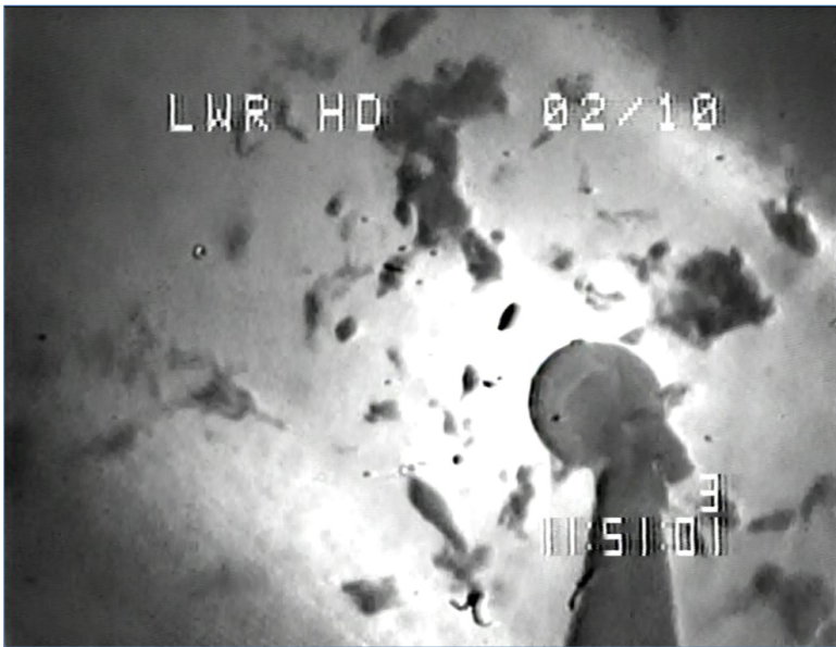
Microorganism growth in the reactor vessel slowed defueling to a halt within a month after defueling started. Shown is the vessel annulus region between the lower core support assembly and the vessel wall.
