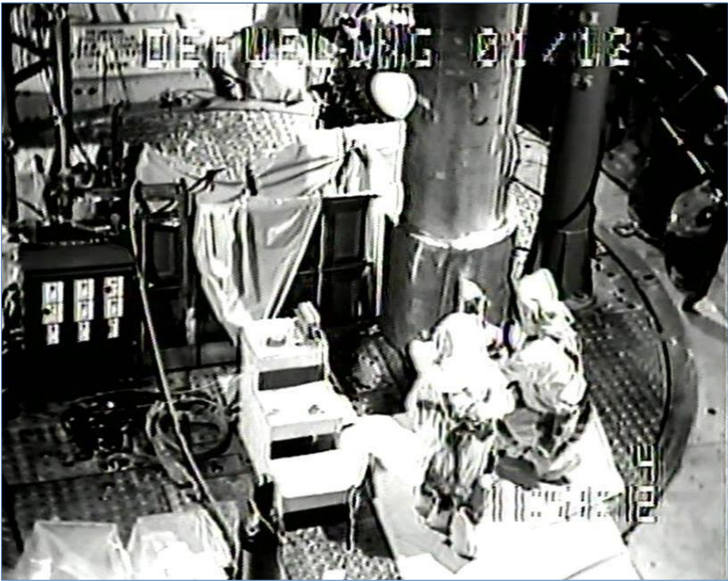
Defueling canister transfer cask positioned over a port hole in the defueling work platform. The canister transfer bridge raised the defueling canister inside the transfer cask, which was then moved to the deep end of the refueling pool.
