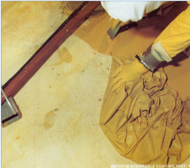
Strippable coating used to decontaminate floor surfaces. (481.15)
