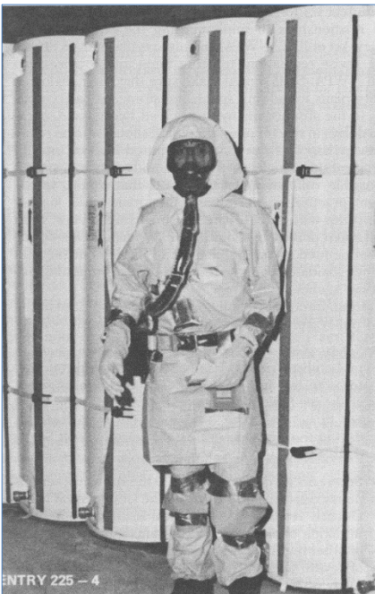
Worker standing next to radiation shielding of interlocking fiberglass columns filled with sand that was used to shield the enclosed stairwell and the reactor vessel head.
