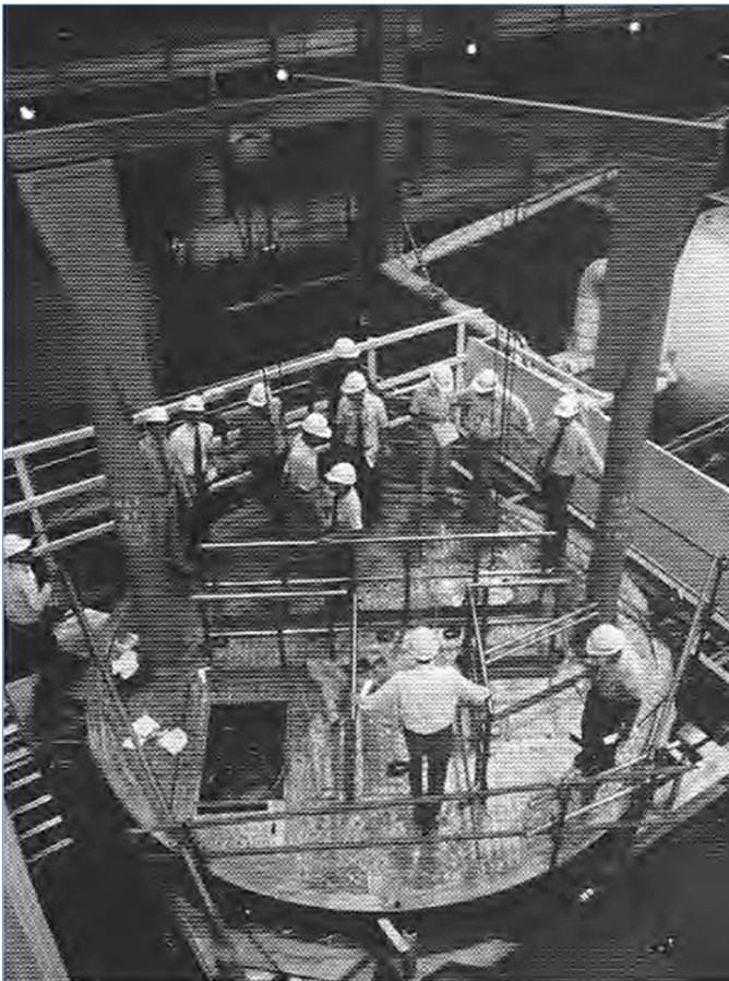
Safety Advisory Board inspecting the mockup in the TMI-2 turbine building of the rotating defueling work platform used to train defueling operators and test new equipment.
