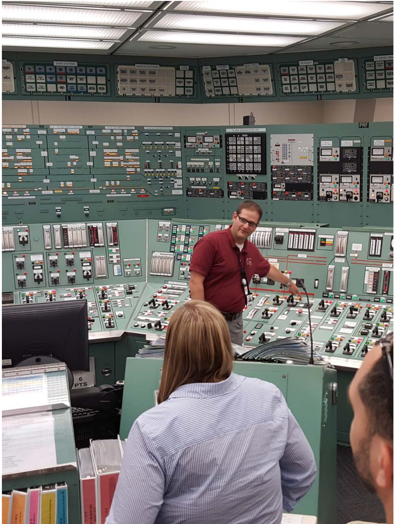
Presentation at Three Mile Island nuclear power plant.
