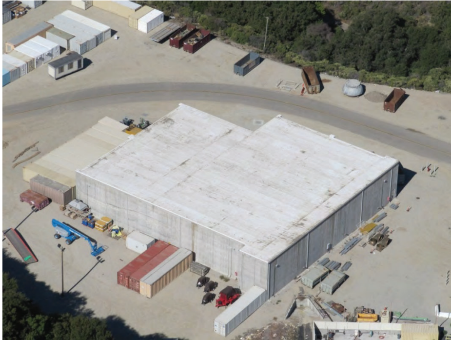
Old Steam Generator Storage Facility looking northwest
