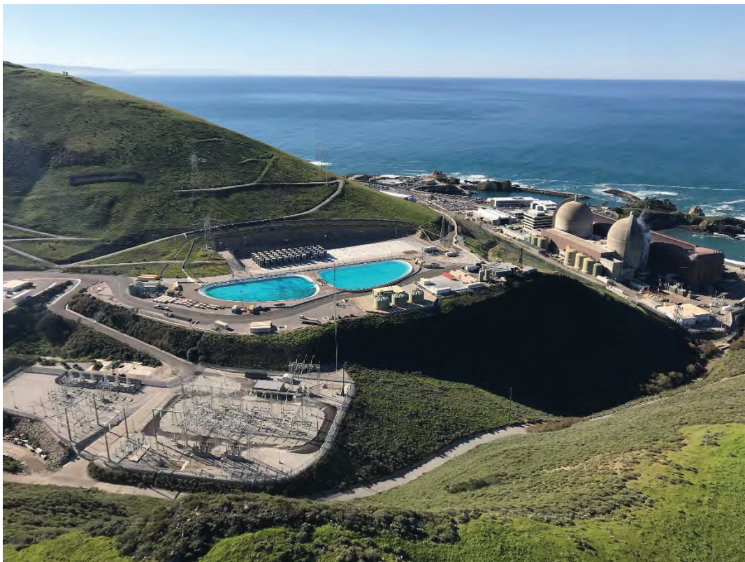
DCPP ISFSI Pad within hillside, on south side of the make-up water reservoirs
