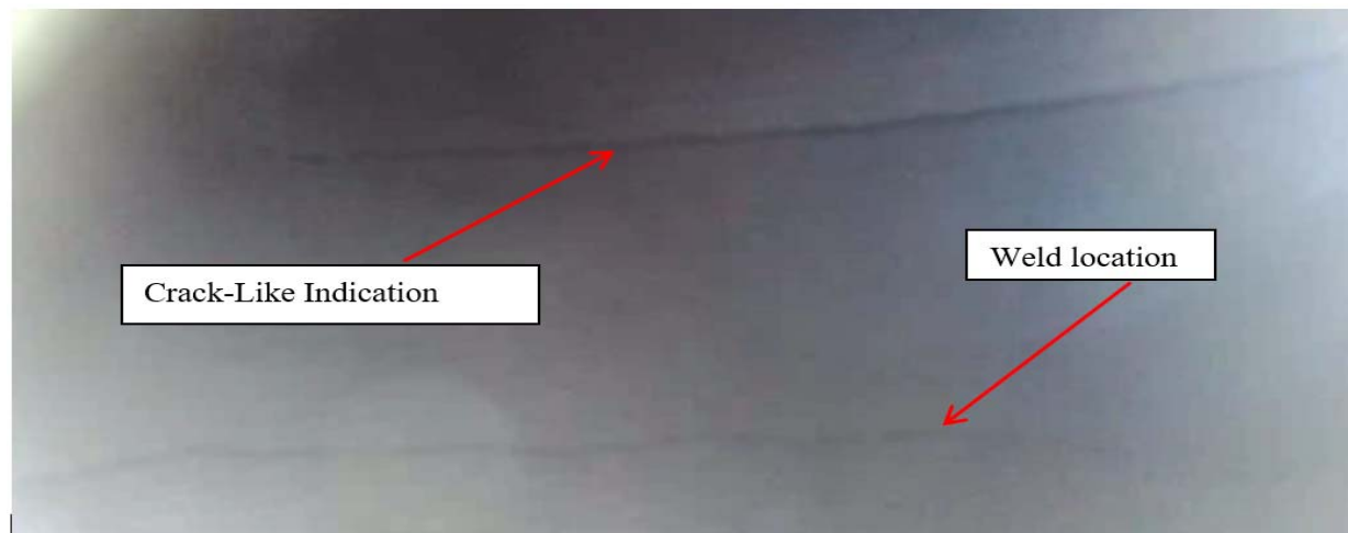
Figure 3 Crack-Like Indication Identified by Visual Inspection
