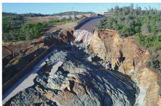
Oroville Dam, Feather River, Oroville, CA 770 feet (tallest embankment dam in US) Spillway Failure February 2017
