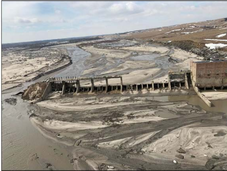
Spencer Dam, Niobrara River, NE (upstream of Gavins Point Dam) March 16, 2019
