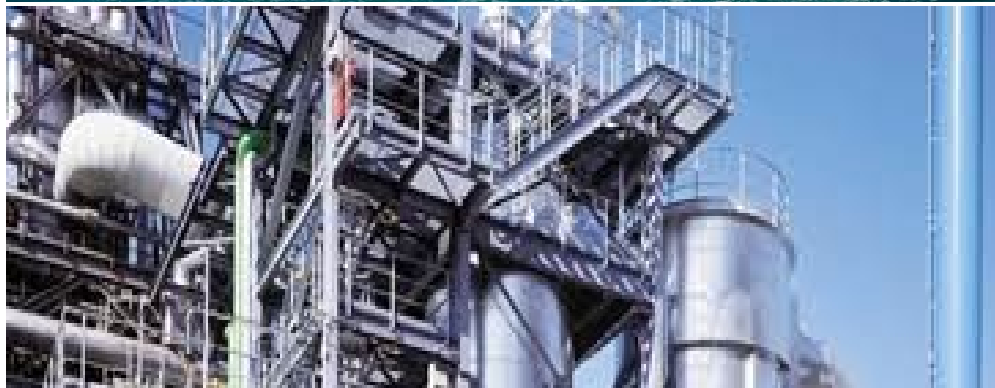
Combined heat and power opportunities at petrochemical facilities worldwide
