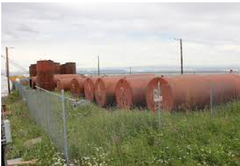
Diesel generator and tank farm in Alaska – opportunities for Micro Reactors in remote areas (including for the US Department of Defense)
