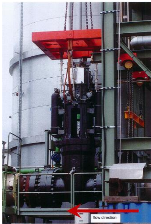
Figure 5: Curtiss-Wright Electro-Hydraulic Operator on MSIV at Karlstein (Source: Author)
