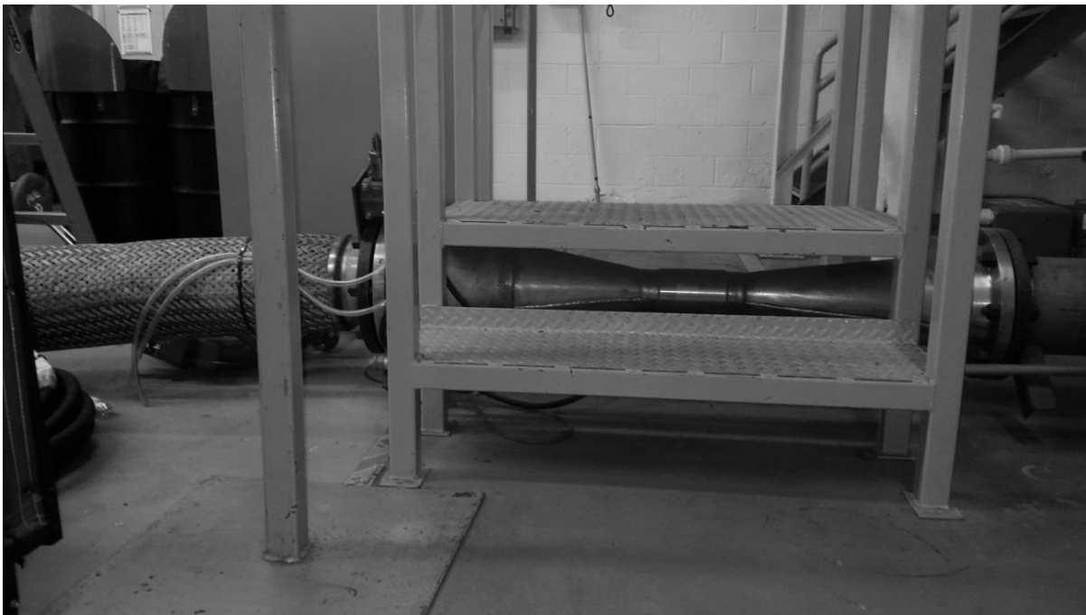
Figure 4. Venturi Meter
