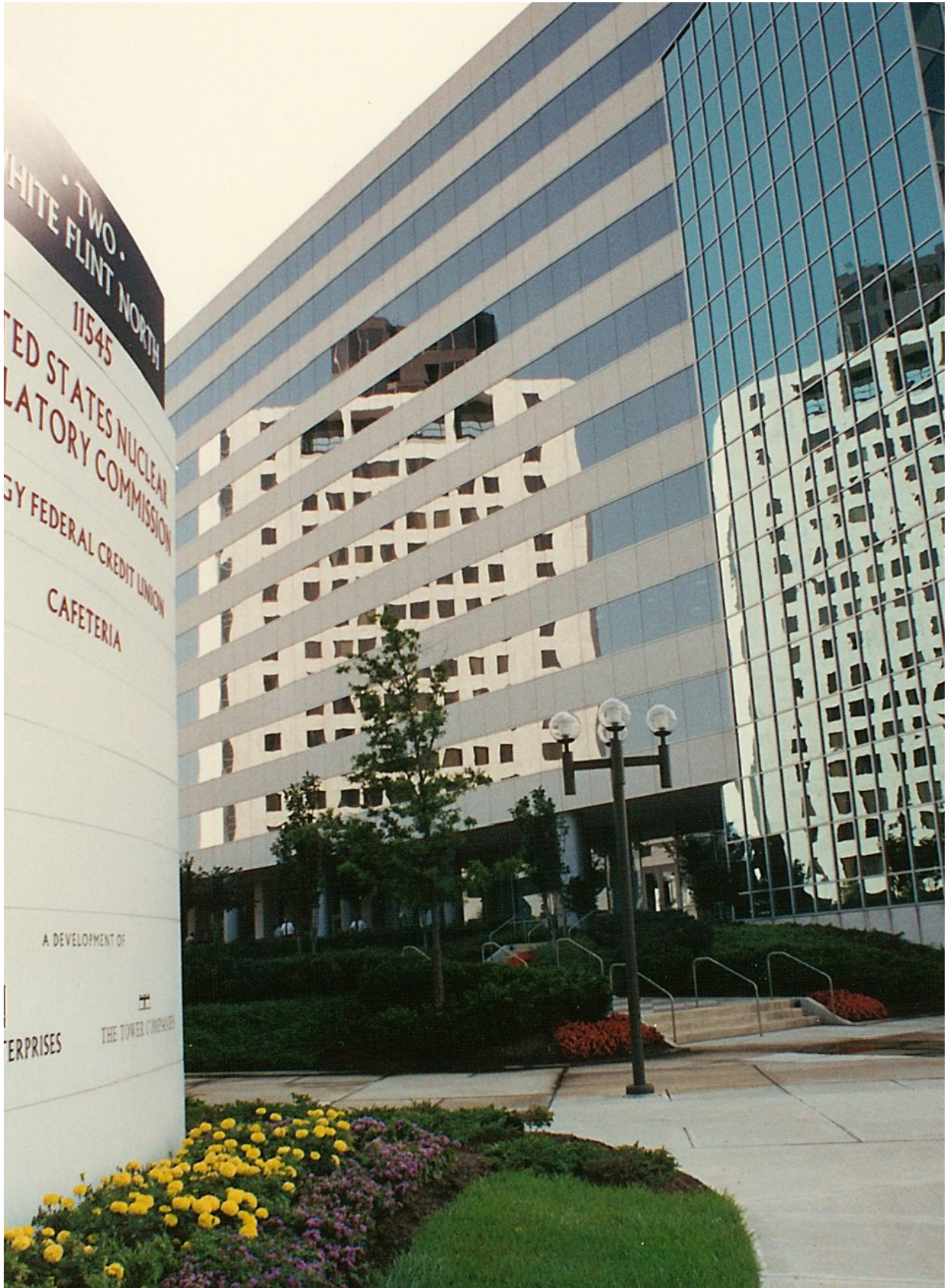
NRC Headquarters complex.
