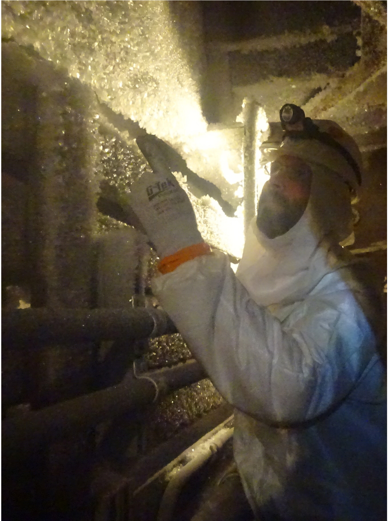
Resident Inspector inspects Watts Bar Unit 1 ice condenser.
