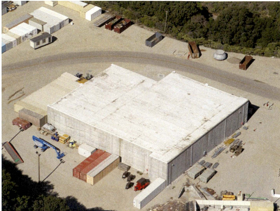
Old Steam Generator Storage Facility looking northwest
