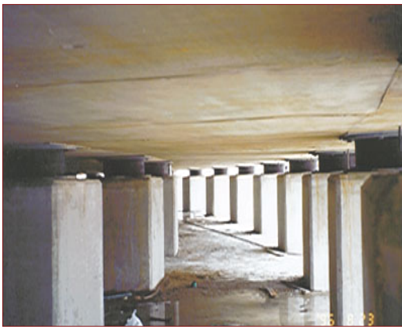
(c) Rubber bearings, Inchon, South Korea
