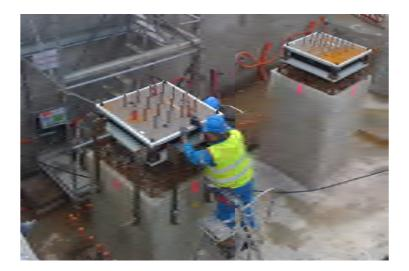
Reactor was isolated using synthetic rubber bearing seismic isolators
