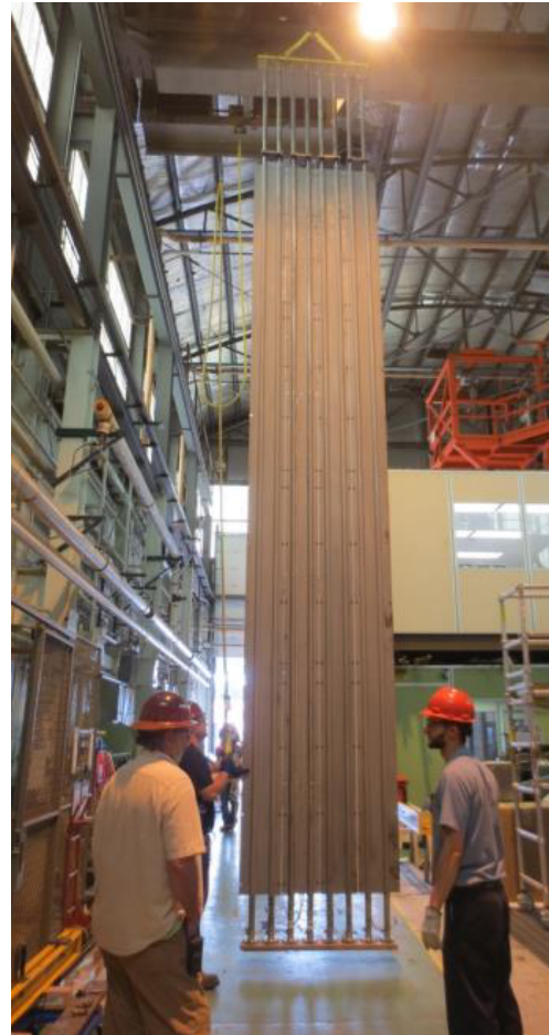
Panel hoisted vertical prior to install
