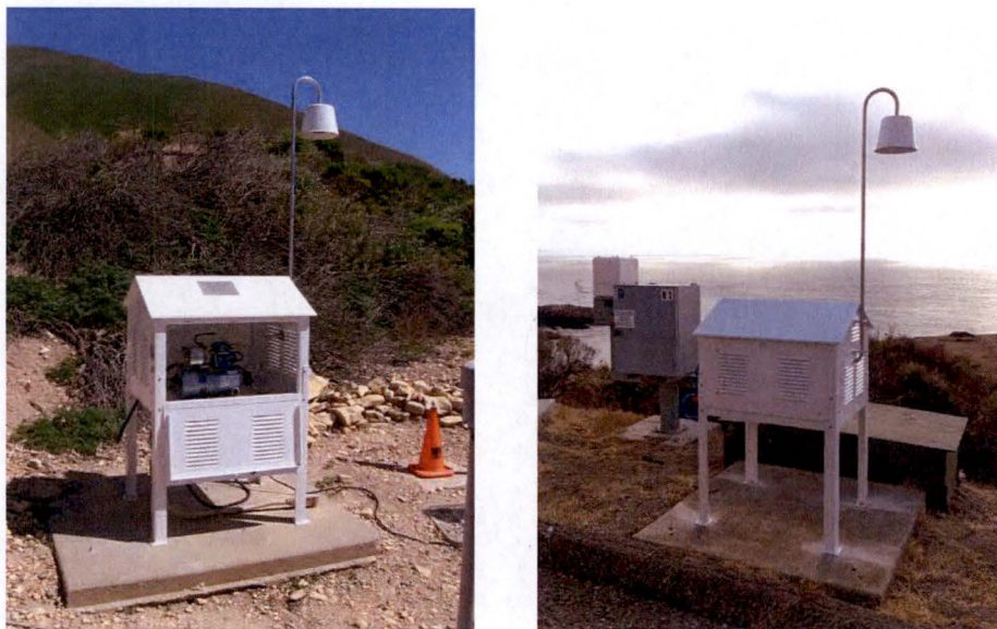
DCPP air sampling station equipment
