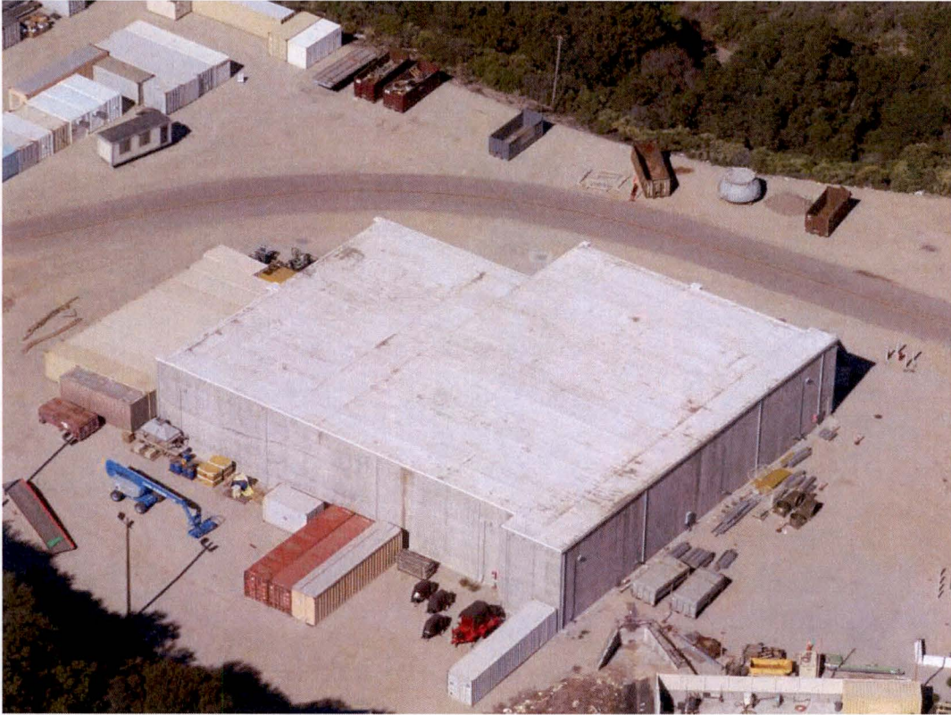
Old Steam Generator Storage Facility looking northwest
