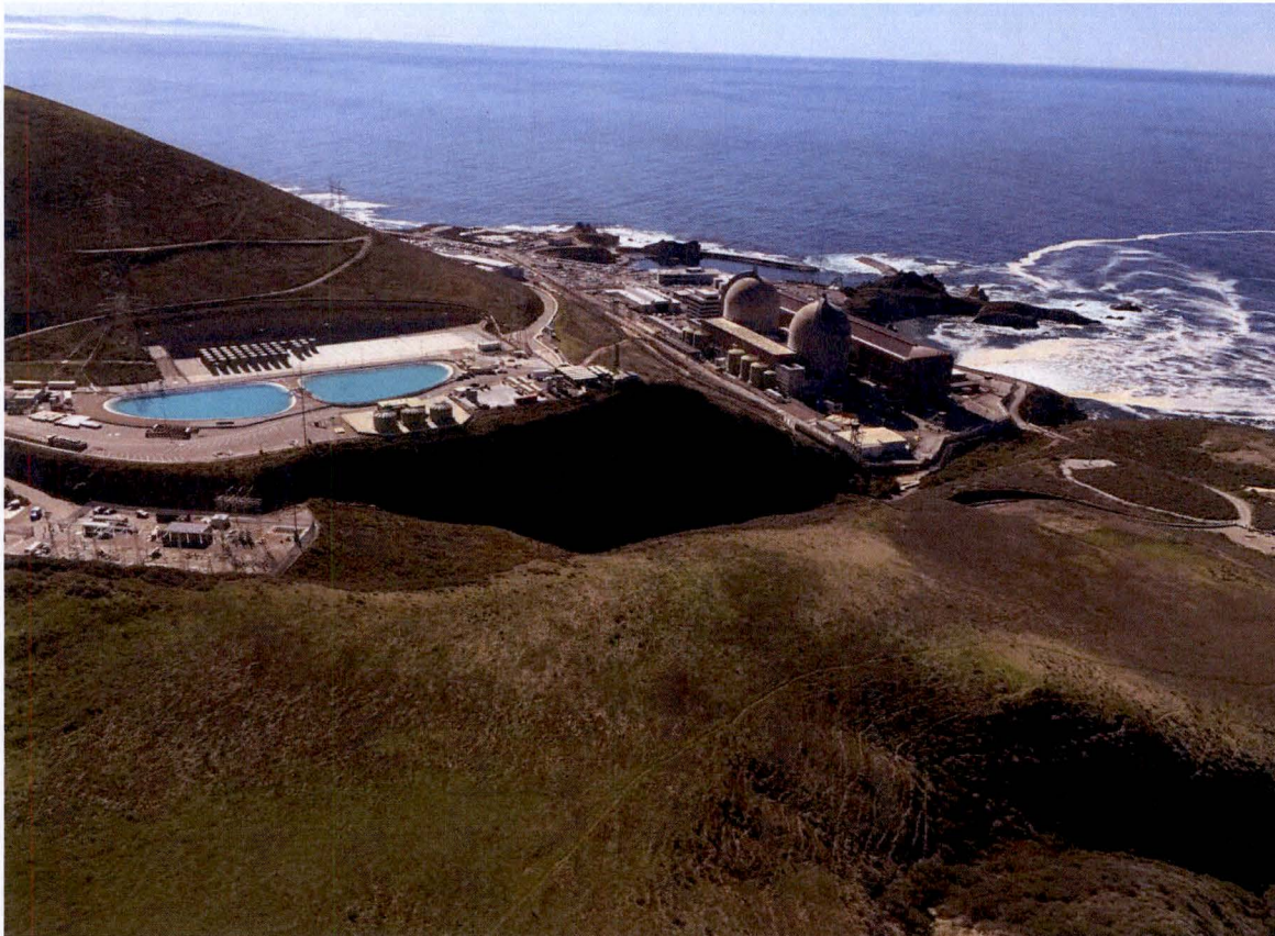
DCPD ISFSI Pad within hillside and south of make-up water reservoirs
