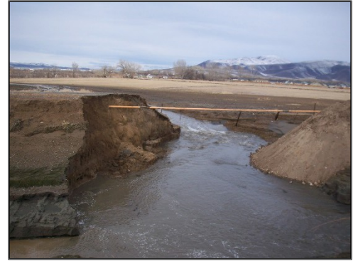
Figure 10.9 Internal Erosion (piping) failure in dam.
