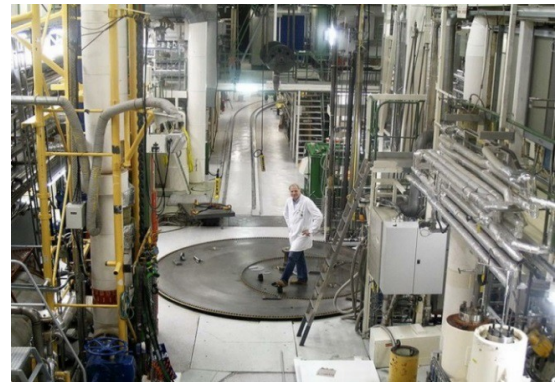
Figure 15.1 Halden Boiling Water Reactor.
