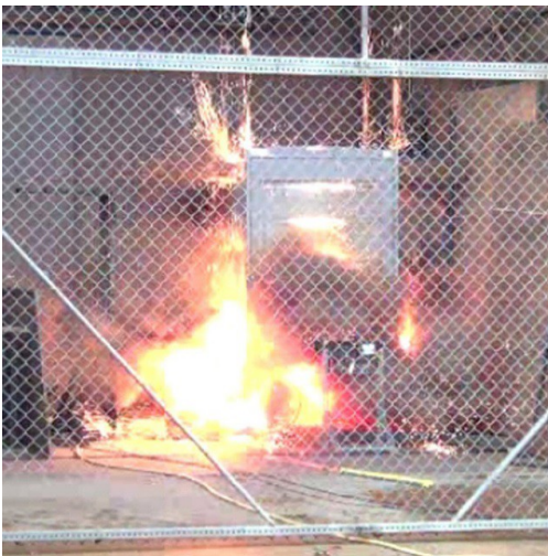
Figure 9.1 Fire Testing of Electrical Components.
