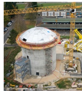
Figure 12.11 Construction of EDF's 1/3-scale PCCV. testing mock up
