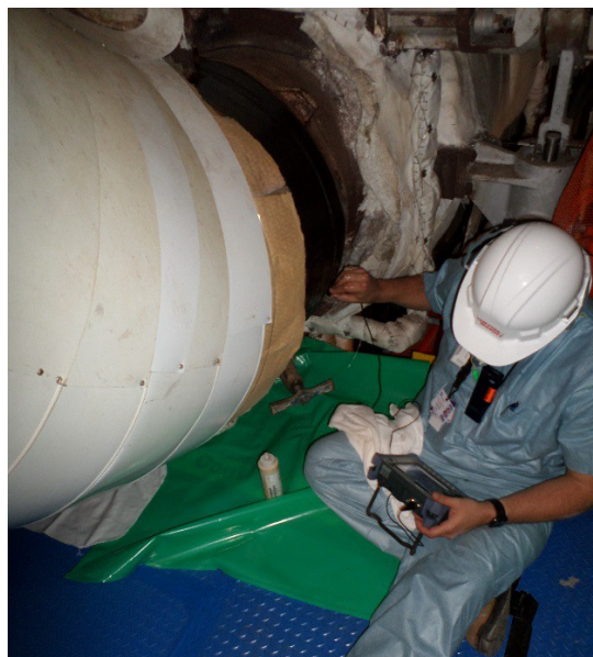
Figure 8.3 Examination of Pipe Weld Using Ultrasonic Testing.
