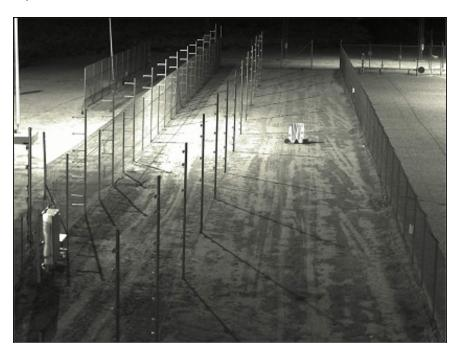
Figure 69 Example of lighting with hot spots, dark areas, and dirt ground cover
