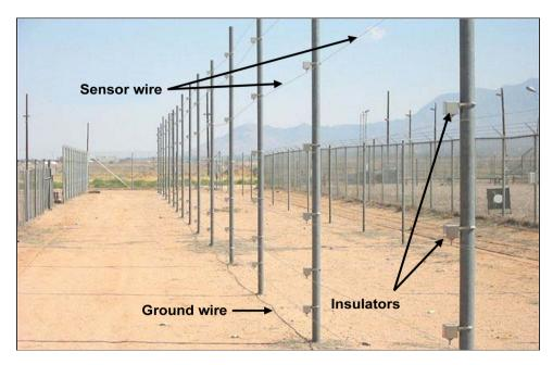
Figure 14 Main components of an electric field sensor installation
