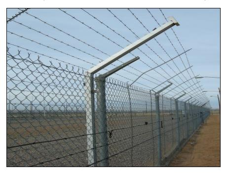
Figure 27 A taut wire sensor system installed on an existing fence
