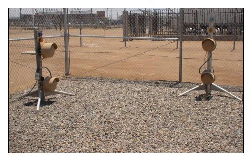
Figure 5 Example of a corner setup of microwave sensors that provides overlap
