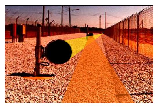
Figure 1 Application of microwave sensors within a PIDAS
