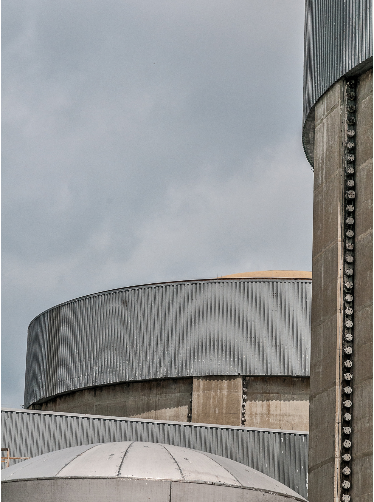
Reactor containment building.
