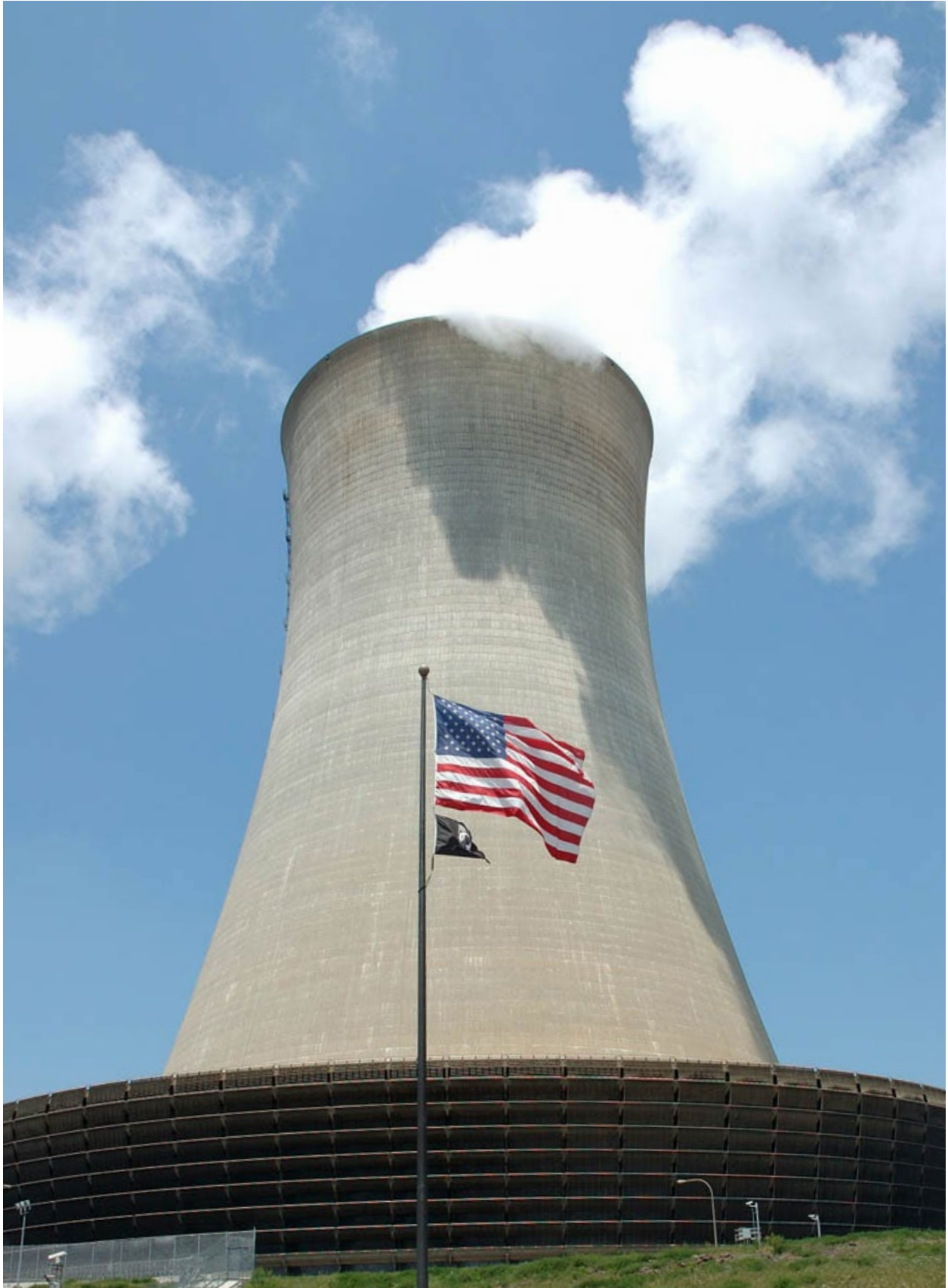
Cooling tower of Limerick Nuclear power plant. Photo courtesy of Exelon Corp.
