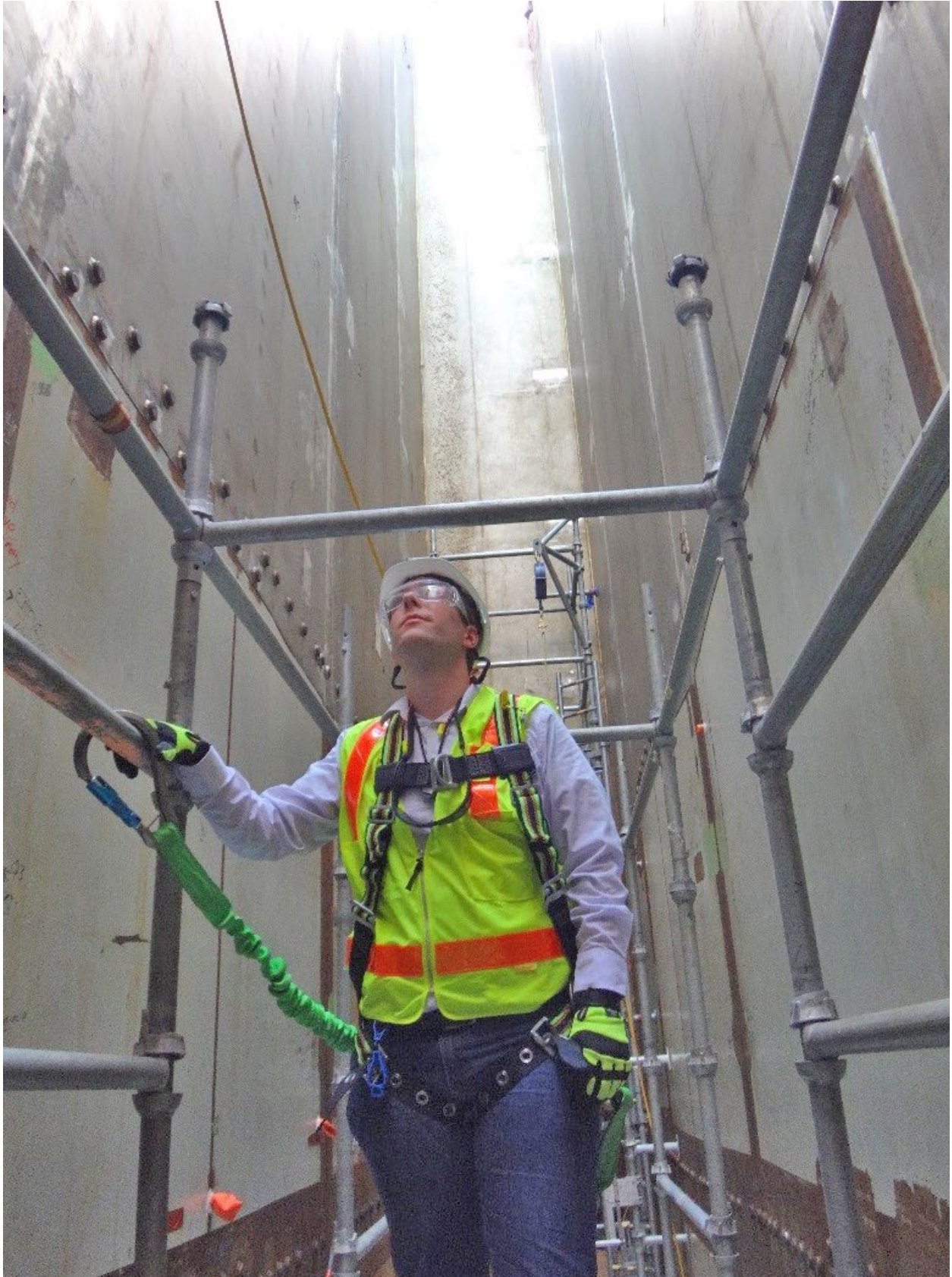
Inspection of construction at V.C. Summer nuclear power station.
