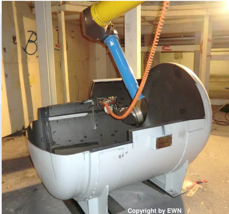
Dismantling of the transfer tank
